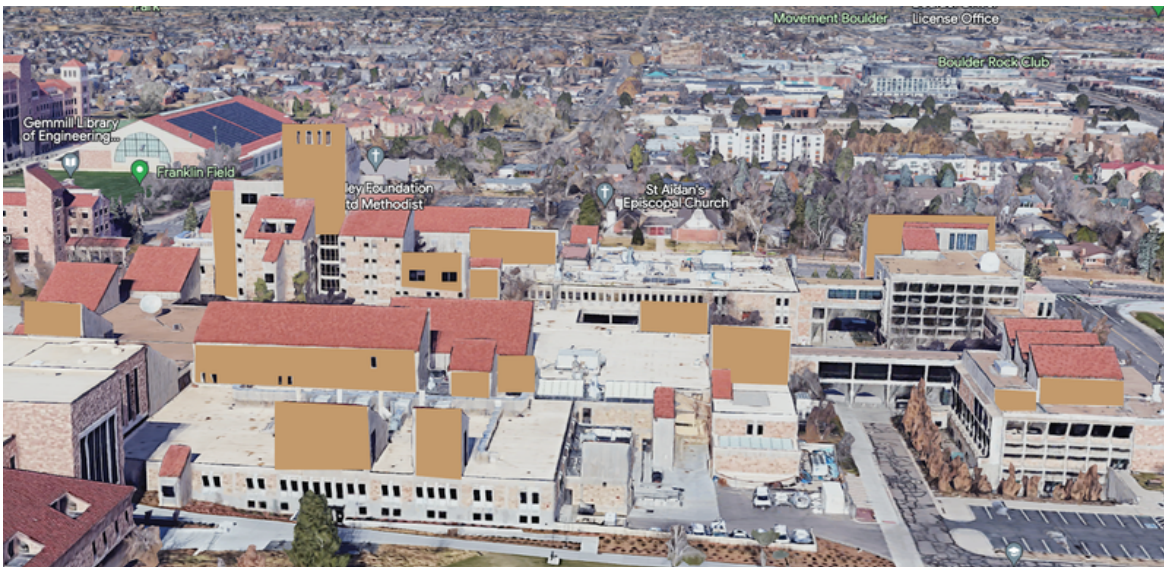
Engineering Center - South facing
