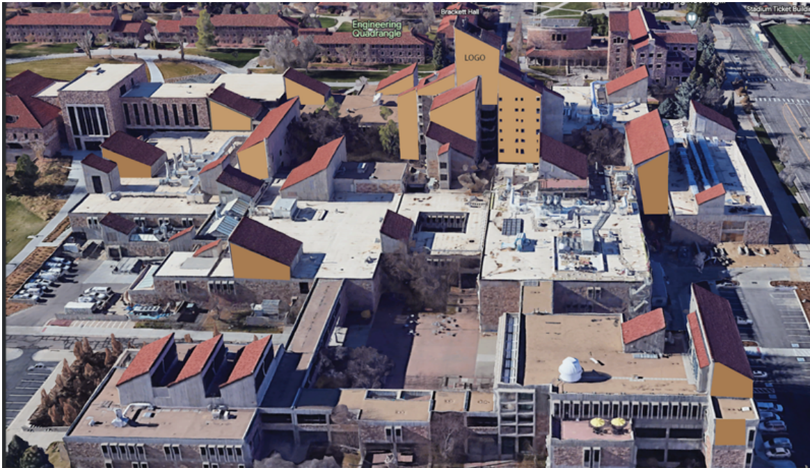
Engineering Center - East facing
